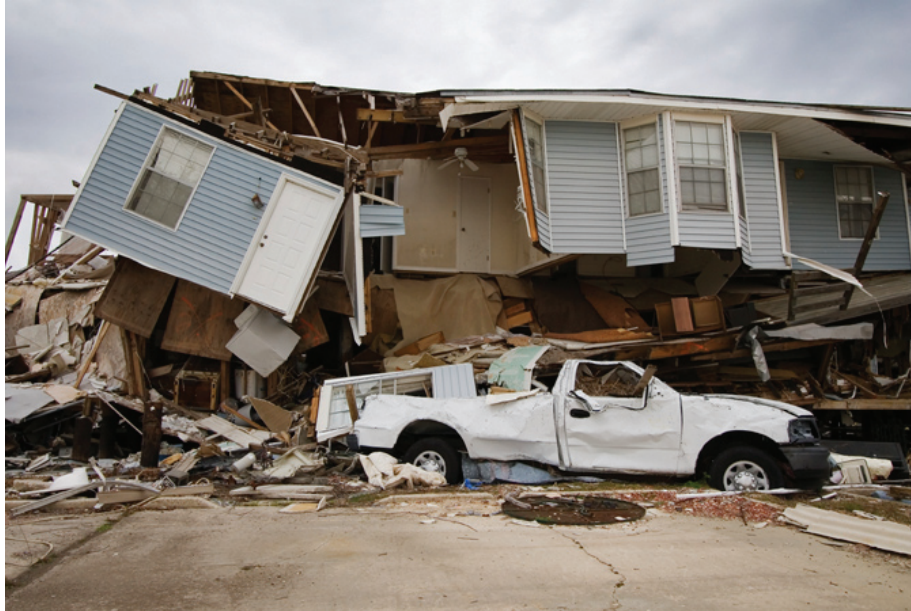
Impact of a Hurricane
